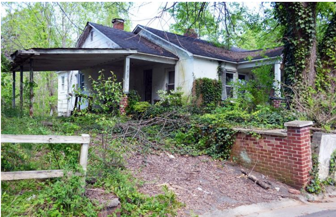
VIRGINIA ANNABLE | NEWS-TOPIC This house on Hillcrest Street is one of many in the West End neighborhood that was left to fall apart after its owners passed away.
